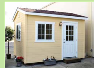
Studio Sheds Built Green
